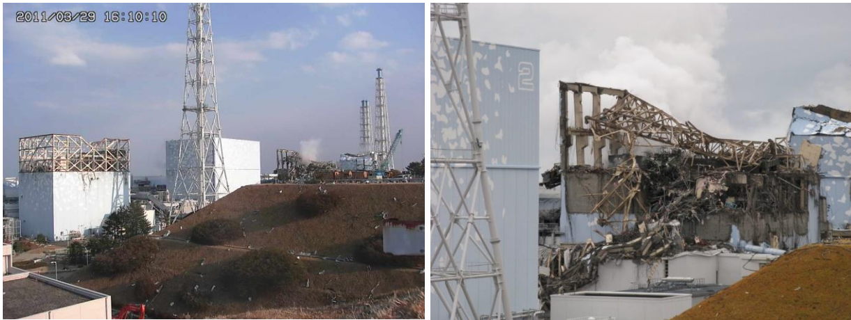
Figure 2-8: Destroyed reactor buildings after hydrogen explosions at the Fukushima Dai-ichi site in March 2011
